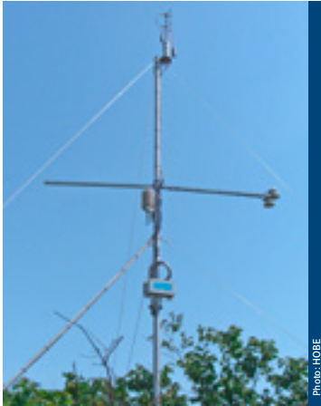
Numerous measuring devices monitor physical, chemical and biological processes
