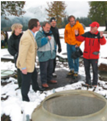
Inspection of the lysimeter network being built in Grasswang
