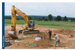
Six additional lysimeters are set up in a circle around every central measurement- and service shaft (top) Once the lysimeters have been set in place and the technology has been installed, the surrounding pit is filled in with soil (bottom)
